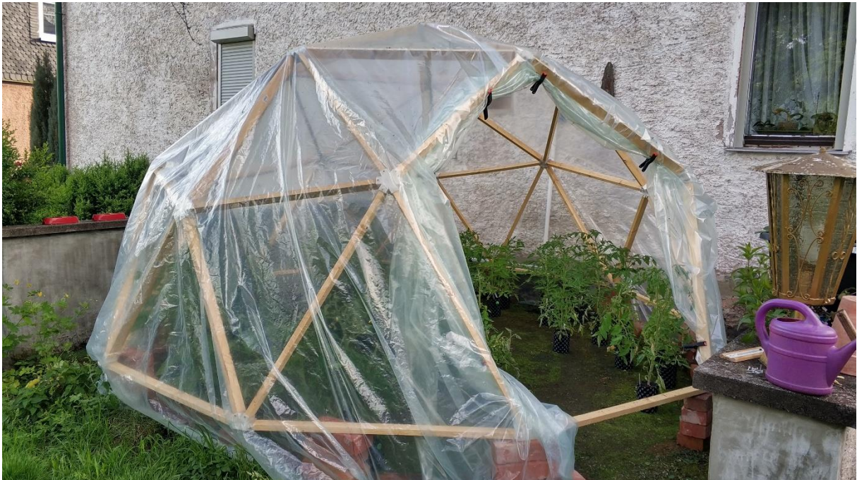
B2: Struts removed for entrance and UV4 greenhouse foil added.
