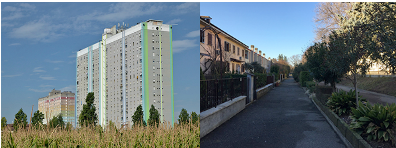
Figure 4 and 5: San Polo Cimabue Tower & residential houses
